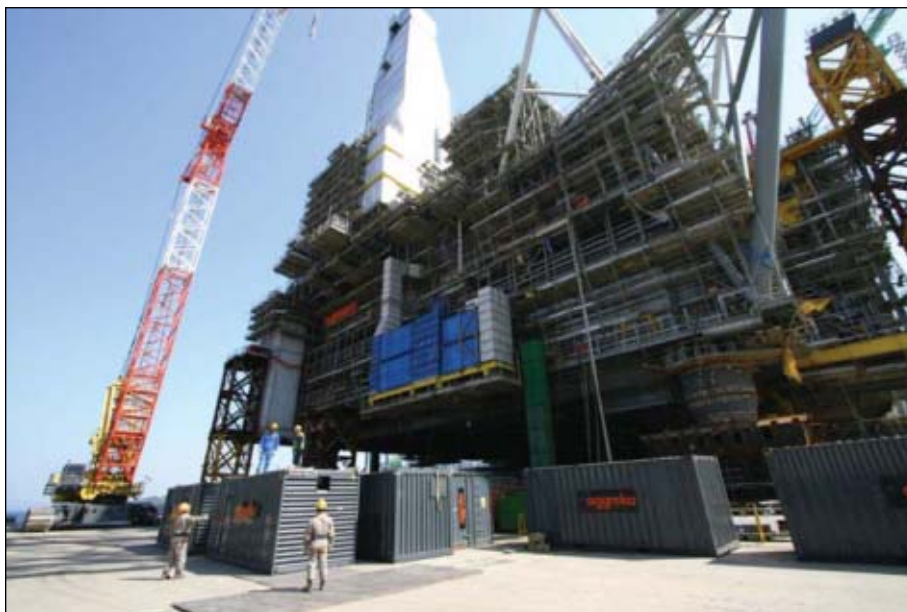
The PA-B topsides needed a turnkey power rental system for the latter stages of the platform's topsides construction and commissioning (Fig. 2). Photo from Aggreko.
